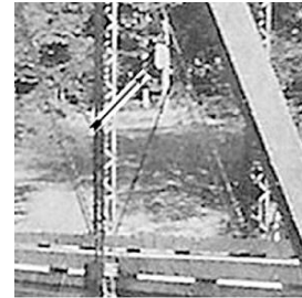
View east at steep entrance
