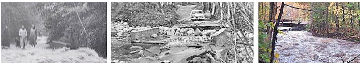
Floods at Culhane Brook Bridge - At left 1954 Hurricane Carol view south courtesy of Paul Shiebler, at center 1959 view north, at right view east at recent close call!
